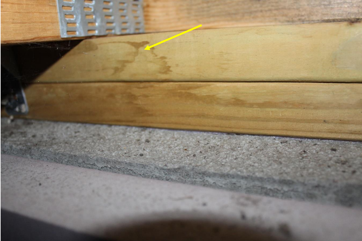
Water stains noticed on the wood framing.
