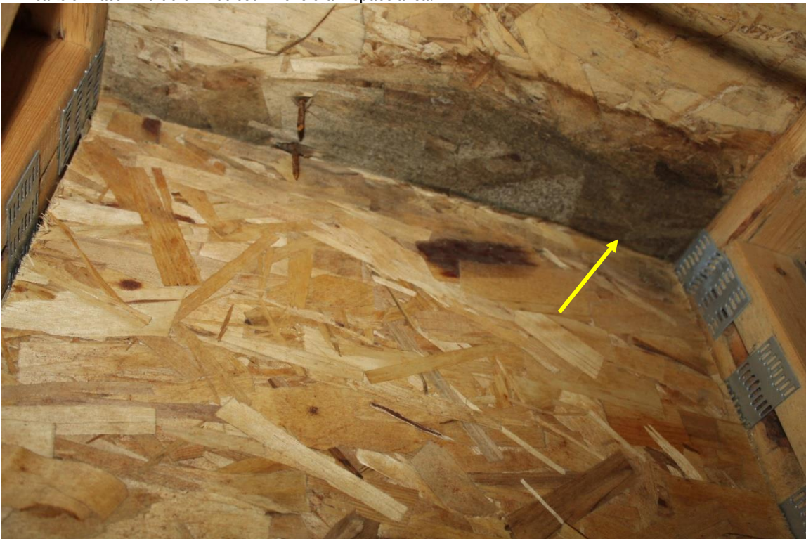
Air leaks & water intrusion noticed in the crawlspace area.
