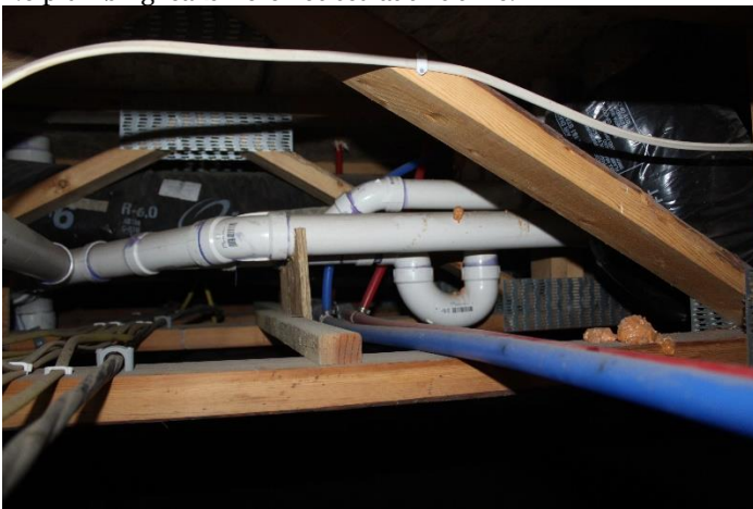
No plumbing leaks were noticed at this time.
