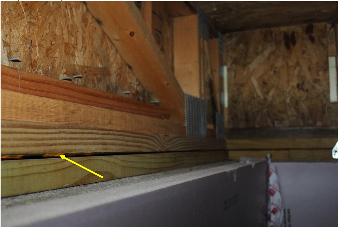
Poorly installed sill plates noticed.
