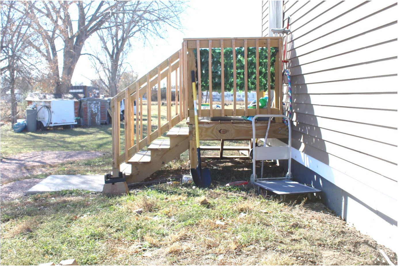
The support posts are resting in the dirt.
