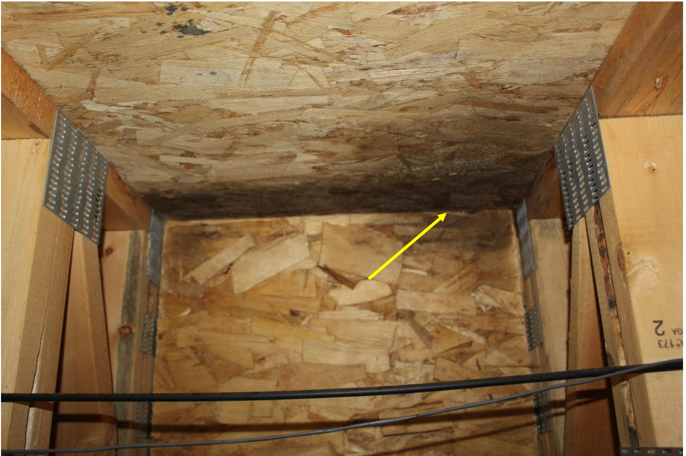
A large amount of spray foam was noticed trying to seal water entry points.
