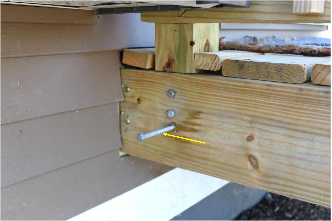
Loose & warped green treated decking noticed. (Missing Fasteners)
