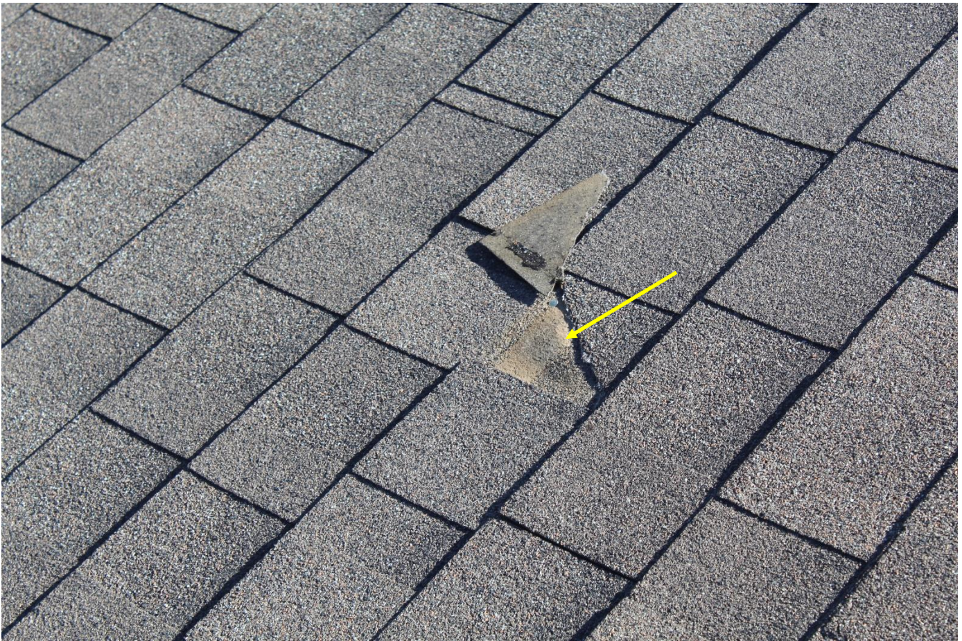
Frayed shingle edges noticed.
