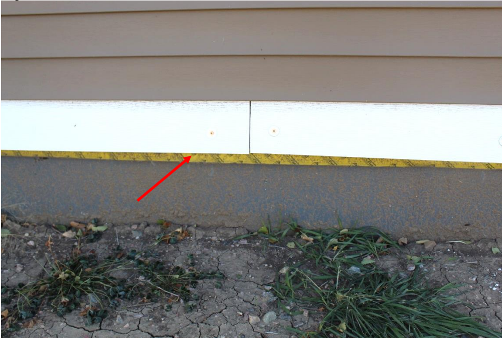
Water entry points noticed behind the siding.
