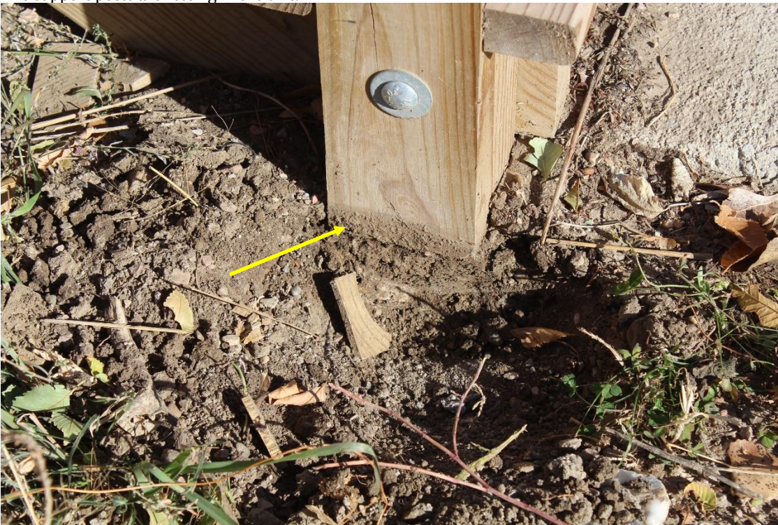
The support posts are resting in the dirt.
