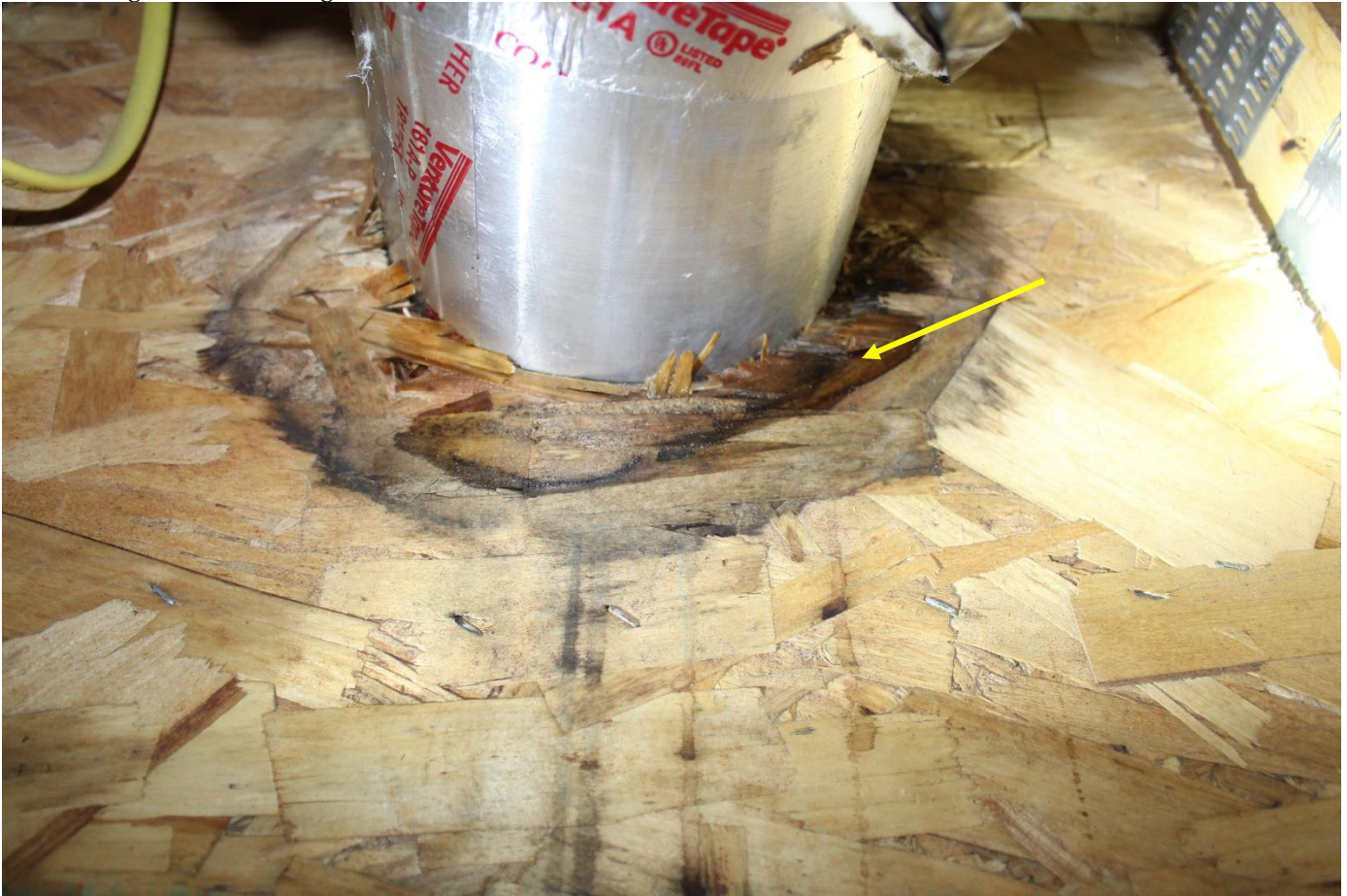
Waterlogged wood sheathing noticed. 100% moisture readings found.
