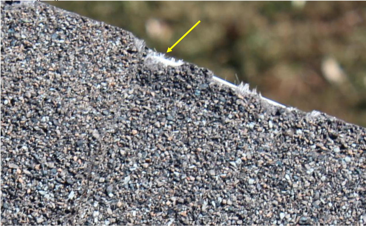
Frayed shingle edges noticed.
