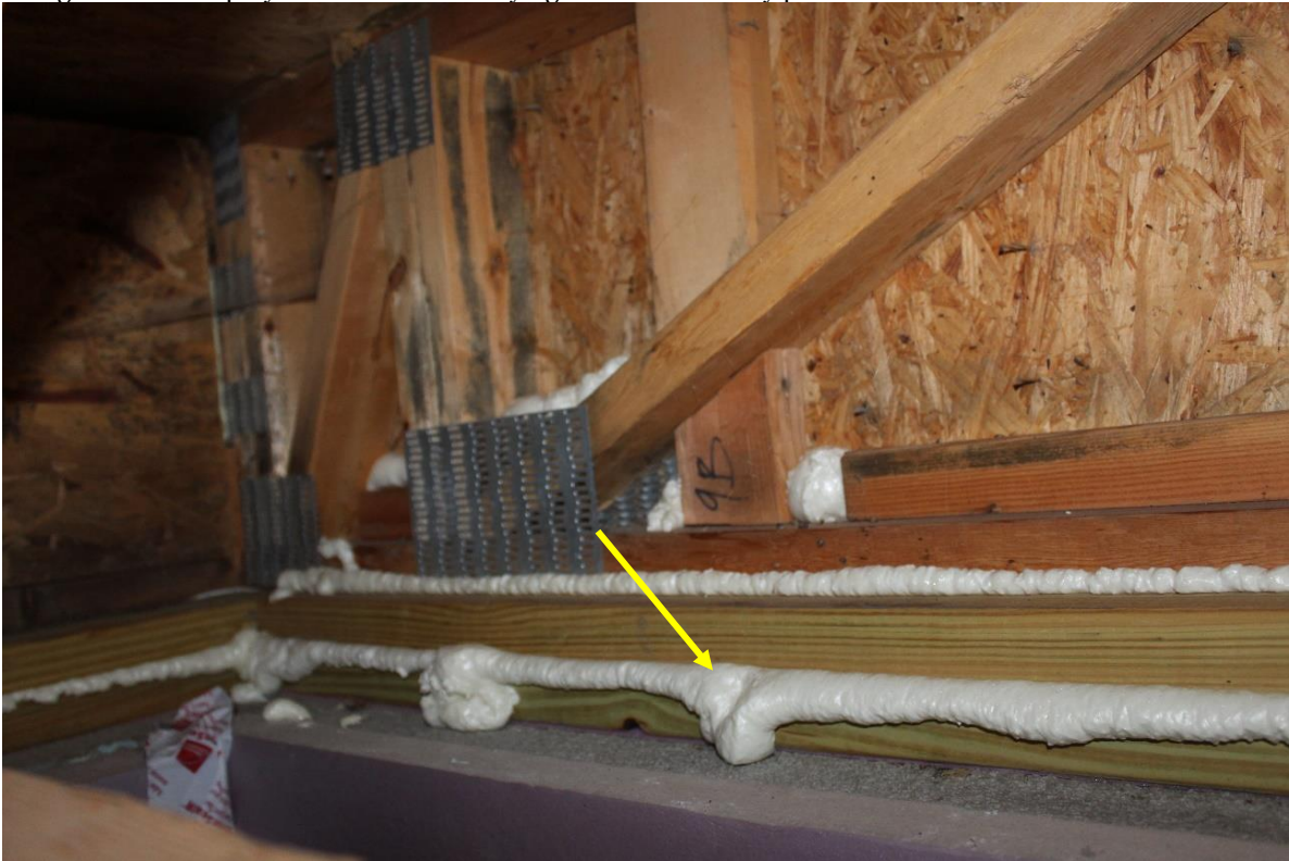
A large amount of spray foam was noticed trying to seal water entry points.
