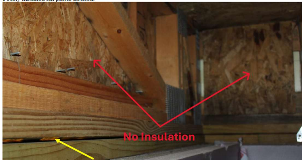
Air leaks noticed throughout the crawlspace.
