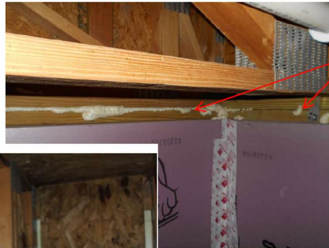
Double Sill Plate on West Wall
